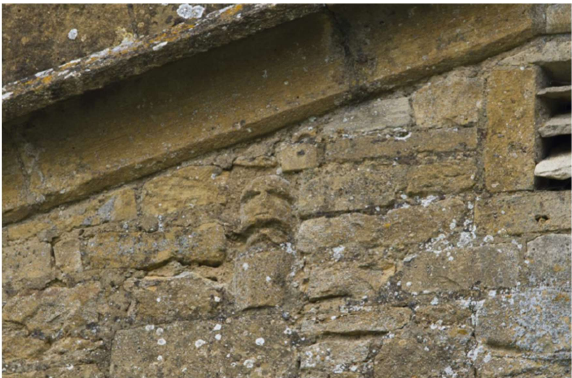
Figure 20: Remnant of possible former column re-set into the western gable end of the church.
